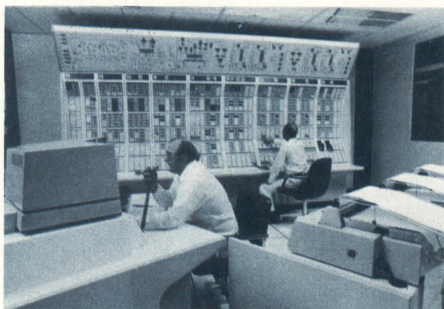
Computer control room. 14' long panel at top of backup panel is complete flow diagram shown in simplified form earlier in this article. Merck designed backup panel can be used for manual control of process if necessary
