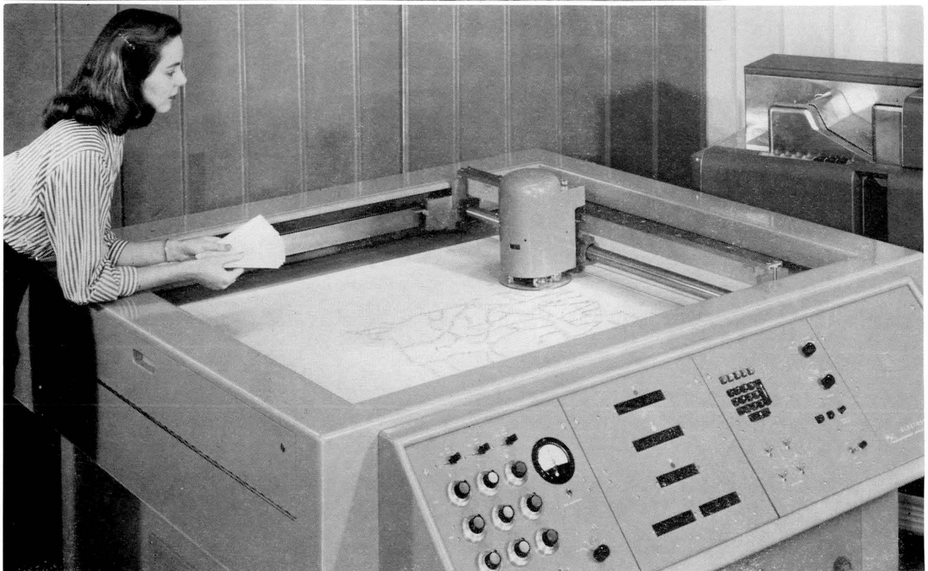
The machine shown above puts out digital and other symbolic displays (eight numbers or symbols printed in parallel) at speeds of up to one display per second. The machine also draws lines. In fact, it can draw any picture consisting of a series of straight lines; for the mapmaker it draws maps; for the highway engineer it draws terrain cross sections and profiles; for the petroleum geophysicist it prints subsurface contours; and for the petroleum production man it presents oil well production information. This machine is the Electroplotter Model S made by Benson Lehner Corp., Los Angeles 64, Calif. (Figure 16)
