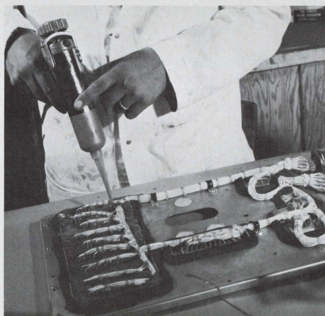
1. Thixotropic high-viscosity epoxy may be applied with an air gun. Epoxy is used as a nonflowing localized embedding material to hold wire to minimize breakage.
