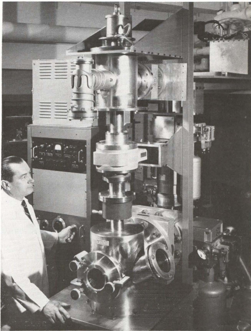
Close-up of an electron/ion and molecular beam unit used in the investigation of selective deposition methods of microcircuits.
