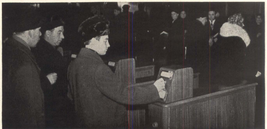
A five-kopeck piece must be inserted first or an electric-eye system will prevent passengers from entering the Moscow metro.
