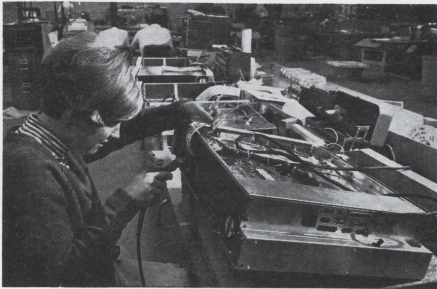
Wrapping it up. Back panel of Data General's Nova computer being wirewrapped. This is final step in chassis construction; p-c boards are then plugged in and machine gets final check.
